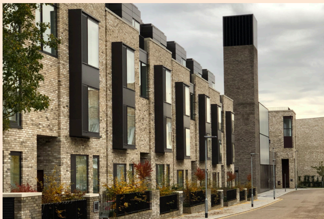
FIGURE 7: ENERGY CENTRE AT EDDINGTON, CAMBRIDGE, WHICH REUSES WASTE HEAT FROM SUPERMARKET FRIDGES TO SUPPLY THE LOCAL AREA WITH HEAT, AND IS INTEGRATED BEHIND SURROUNDING HOMES
