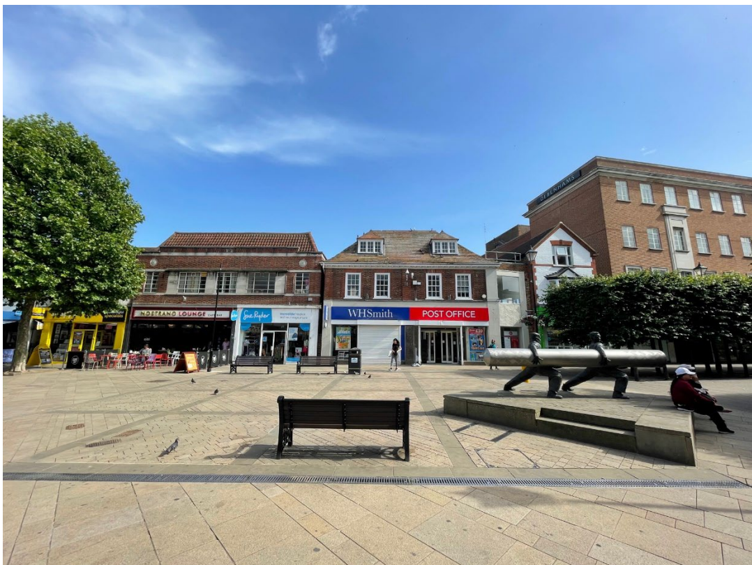
Plate 2 Looking south to 47-57 High Street
