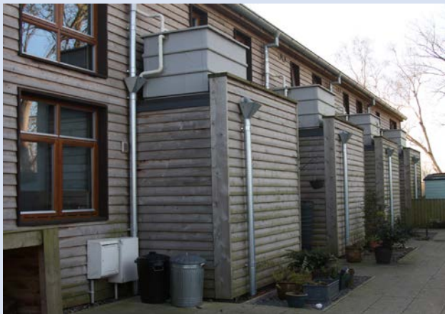
FIGURE 25: HOME RAINWATER CAPTURE SYSTEMS
